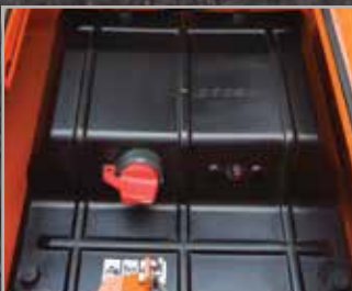
Battery cut-off switch
