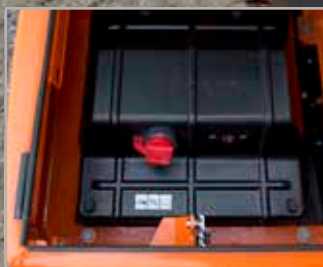
Battery cut-off switch
