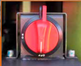
Battery cut-off switch
